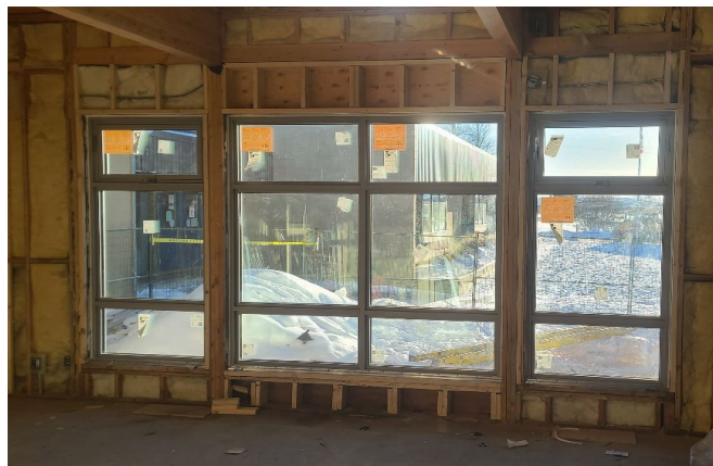
New windows looking South from Group A and Group B rooms
