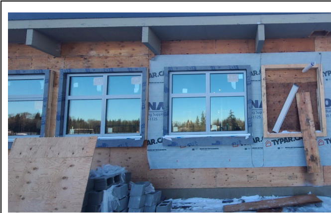
Installation Progress on N side
