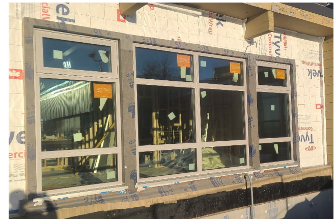
New windows from the outside
