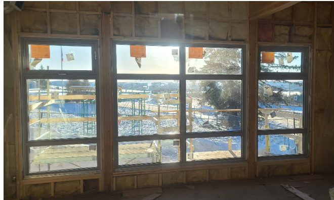
New windows looking South from Group A and Group B rooms
