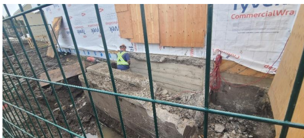
The library foundation was removed to allow for the drain tile installation and eventually new sidewalk
