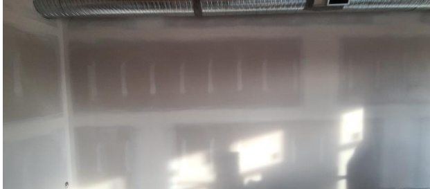
Inside, Drywall, Mud & Taping is completed
