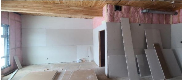
Drywall being installed over the insulation and electrical / plumbing rough ins.
