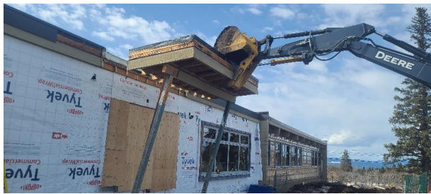
The old library entrance canopy was removed.
