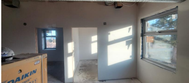
Foods Classroom with primer coat
