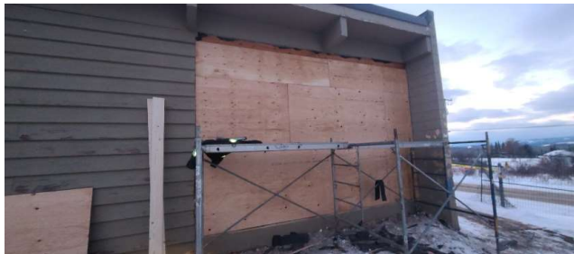
Closed up from the outside with new sheathing
