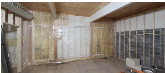
More New window framing for large windows on the S side.
