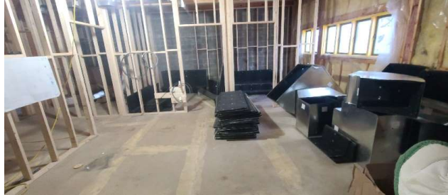
Meanwhile, Inside the HVAC and Plumbing was being installed.
