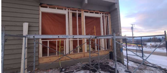
New Window sizes on the N side of the building
