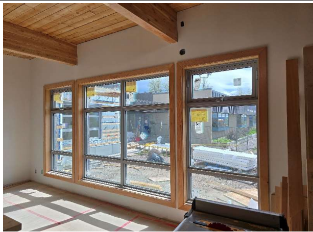
Finished windows in the 3-5 yr old daycare room
