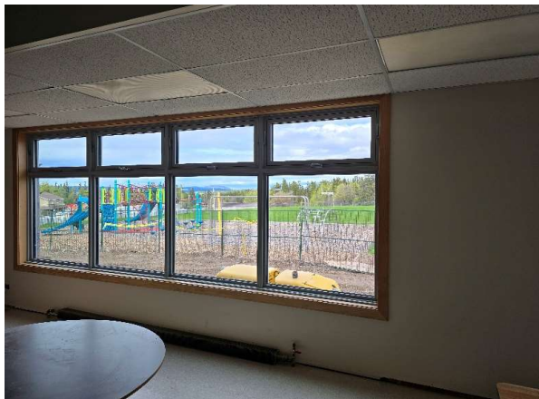
Fir window trim was installed and the walls painted in the library
