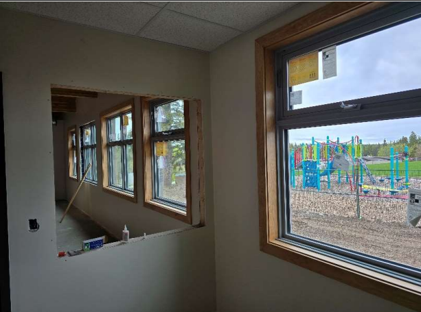
Lots of finishing work going on inside
