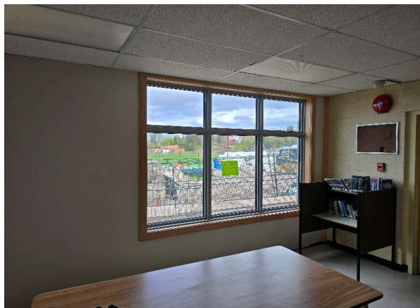
The library window where an old door used to be, trimmed out and painted
