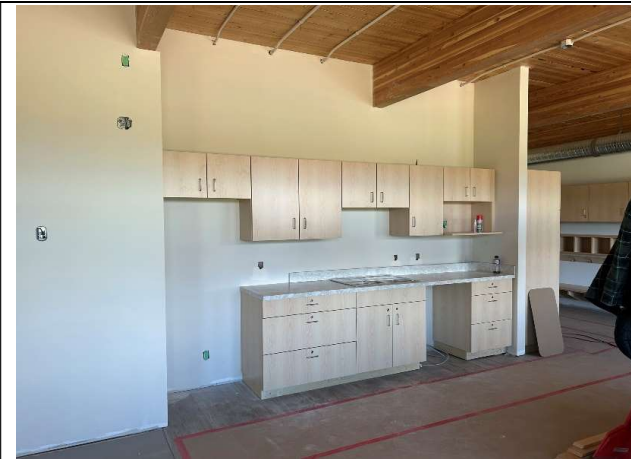
Cabinetry is being installed in all of the rooms
